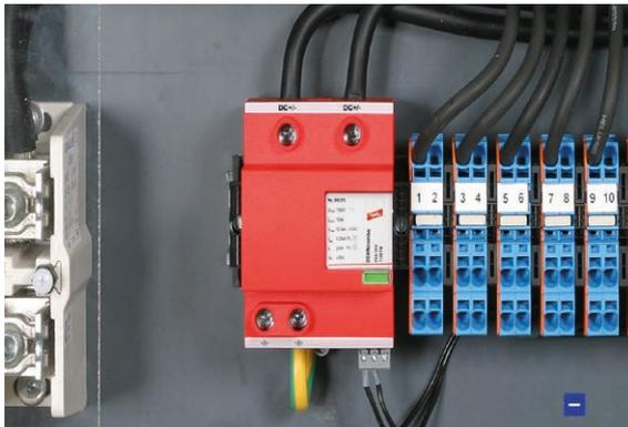
Figure 6 DEHCombo YPV type 1 combined arrester for protecting photovoltaic systems from surges and partial lightning currents
