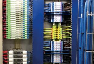
Optimum protection of control and telecontrol systems with a coordinated surge protection concept
