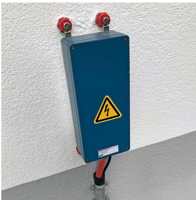
Coaxial connection box with integrated EXFS 100 ex isolating spark gap
