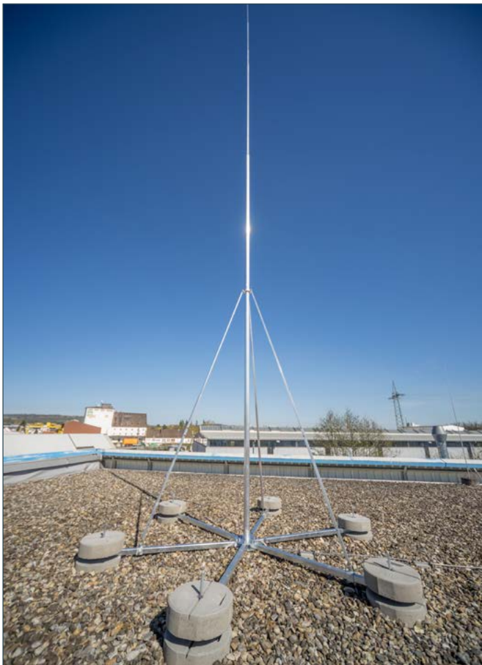
Ball joint mounted adapter between the two base plates of the six-legged stand.
